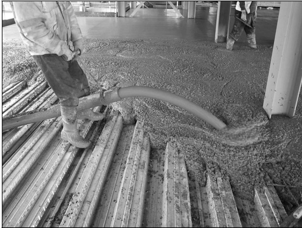
Figure 6.4 Pumping of fibre-reinforced concrete
