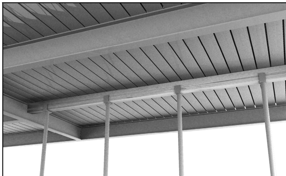
Figure 4.17 Temporary support using an 'Acrow' props
