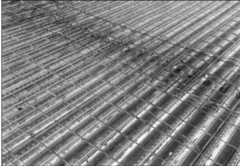
Figure 6.3 Decking and fabric reinforcement – ready for casting the concrete
